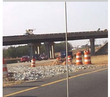
US 70 construction in Johnston County
